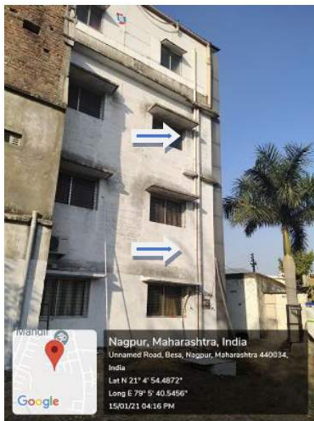
Pipeline to flow harvested rain water to soak pit
