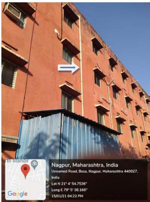
Pipeline to flow harvested rain water to tanks
