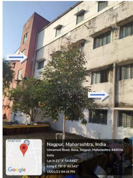
Pipeline to flow harvested rain water to soak pit
